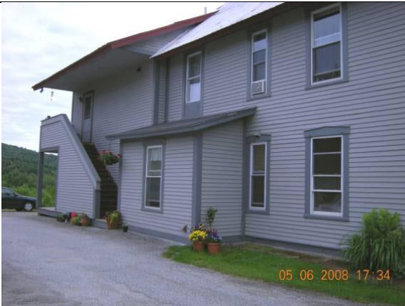
View to laundry and steps to apt 4
